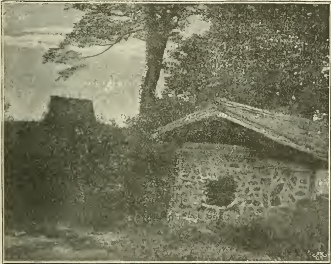
BEACON TOWER ON NAM SAN
